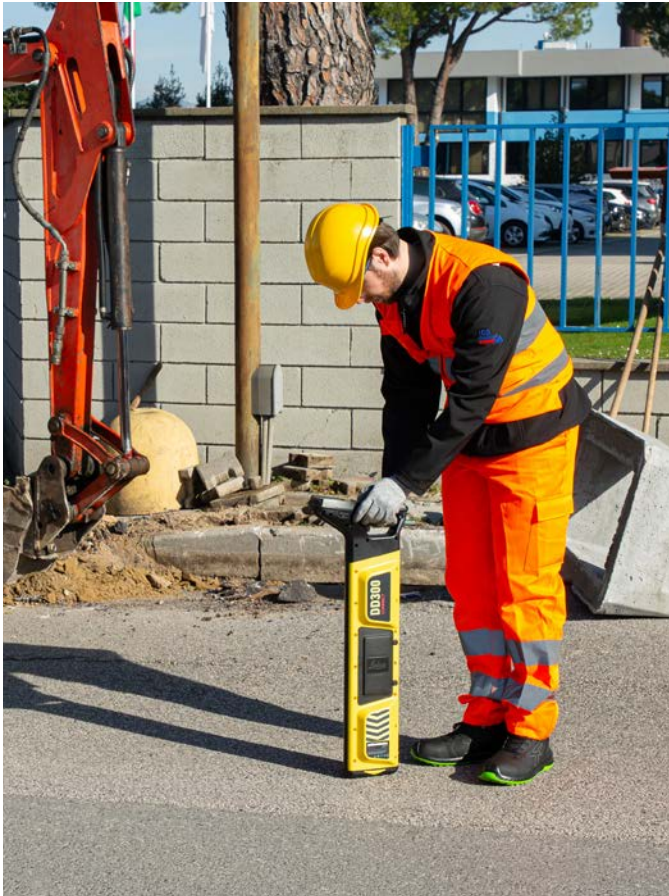
* Pipe energized with Signal Transmitter
